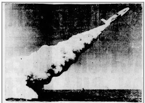
BLASTING OFF amid cloud of smoke from its jet assisted takeoff bottles, Navy's surface-to-surface guided missile Regulus leaves launching platform aboard the submarine Tunny during operations off the California coast.
